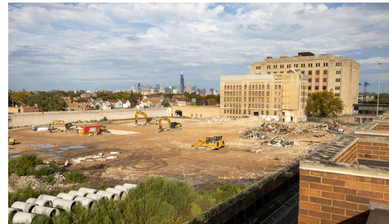
Demolition of Divisions I and IA at the Cook County Jail
